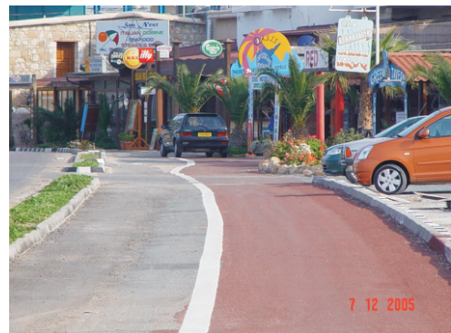
Figure 2: Application of red slurry seal at Latchi, Pafos
