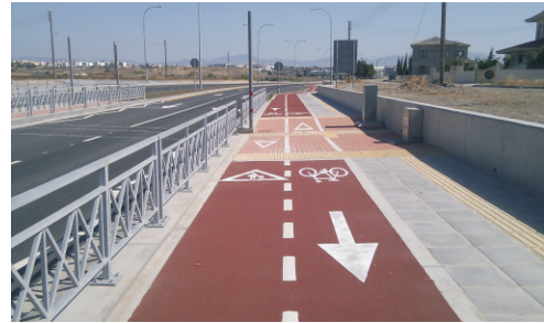
Figure 4: Application of red slurry seal at G.S.P.,Nicosia
