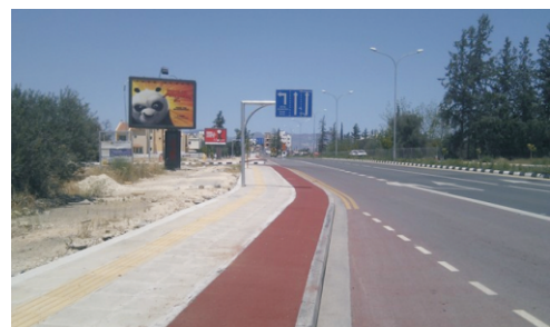
Figure 3: Application of red slurry seal at Egkomi, Nicosia
