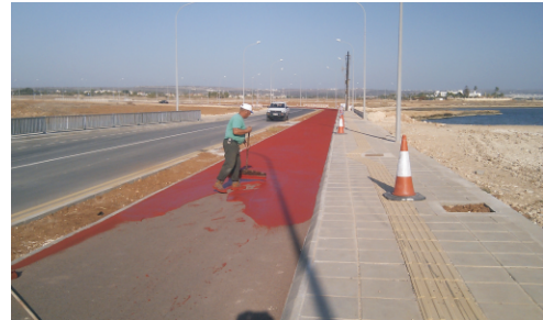
Figure 1: Application of red slurry seal at Agia Napa
