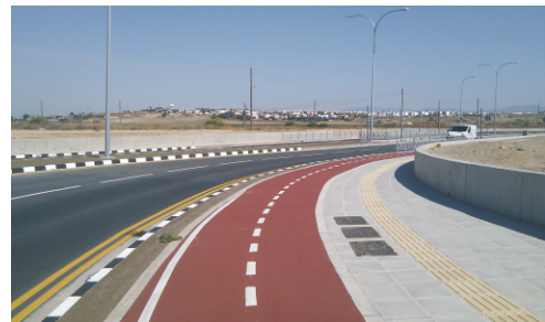
Figure 5: Application of red slurry seal at G.S.P.,Nicosia
